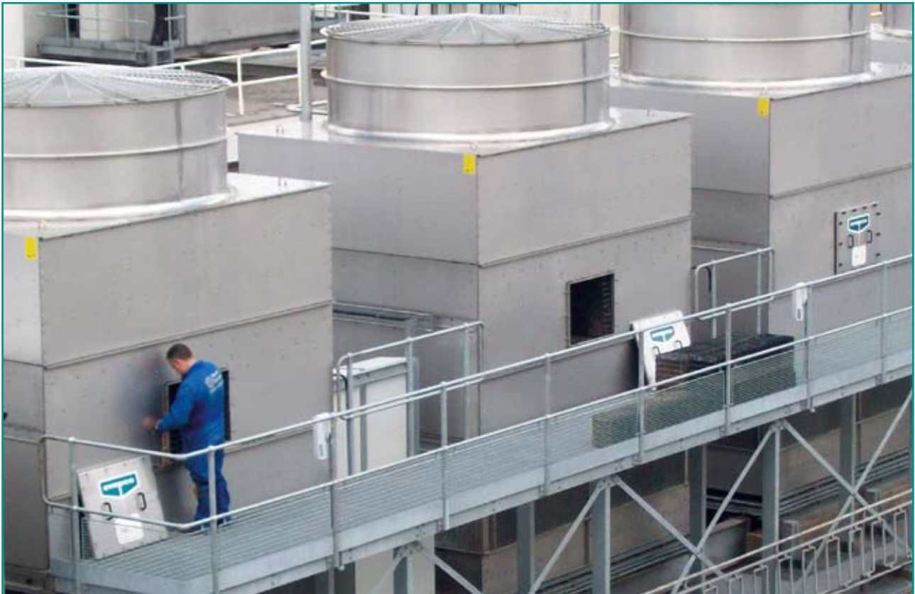
Custom design platform to enable inspection and periodic removal of fill pack
