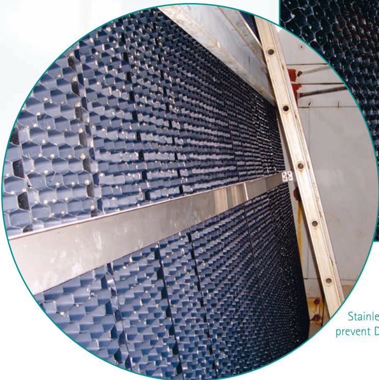
Fill pack is lightweight and easily installed/removed by one man
