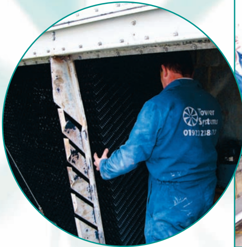
Fill pack is lightweight and easily installed/removed by one man
